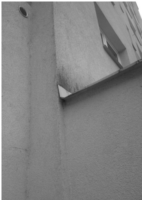
Fig. 1. Part of the roof construction and piping
