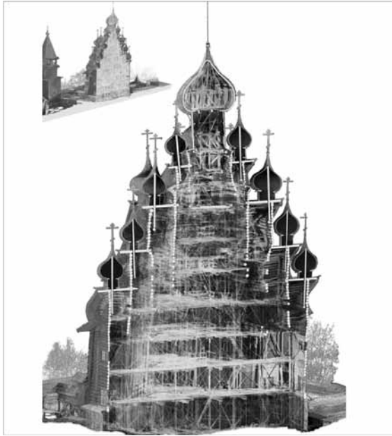
Fig. 2 The project concerns the Pogost complex, with a detailed and accurate analysis of the architectural and static structure of the Church of Transfiguration for the study of conservative and restorative methodologies. The project focuses on general survey of the object through different methods: laser scanner survey, direct survey, general analysis, realization of a wide photographic campaign and detailed drawings analyzing from the general to the detail. The results consist in 2D and 3D drawings, digital databases, census archive and 3D reconstructions.
