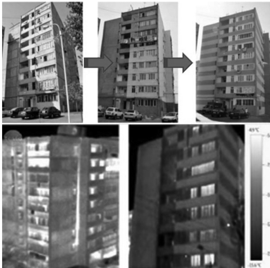
Fig. 2 Large panel building renovation in Avan district/ infrared .view of building( before-after)
