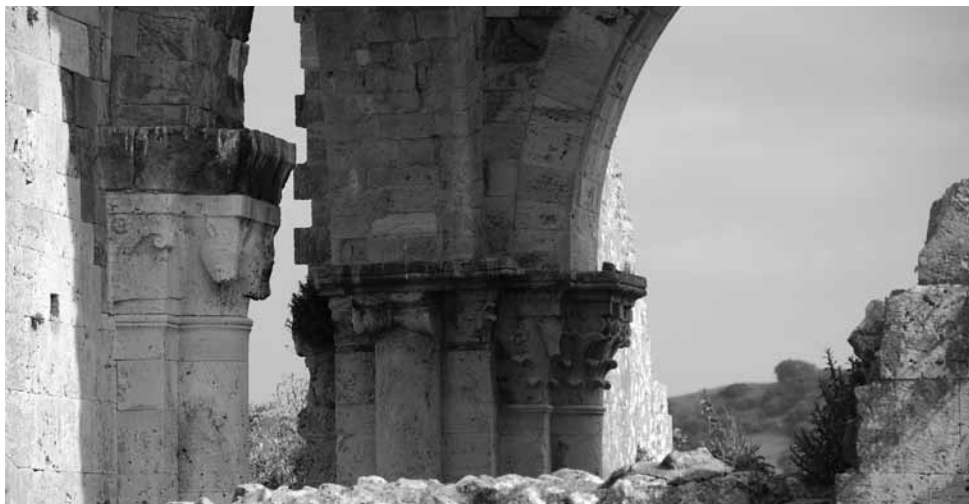
Fig. 3 Picture of some capitals with Romanesque refined decoration depicting animal figures and foliage. One can note the different coloring of the stone material. Featured remnants of the cladding wall on the south side where we can see the typical wall.
