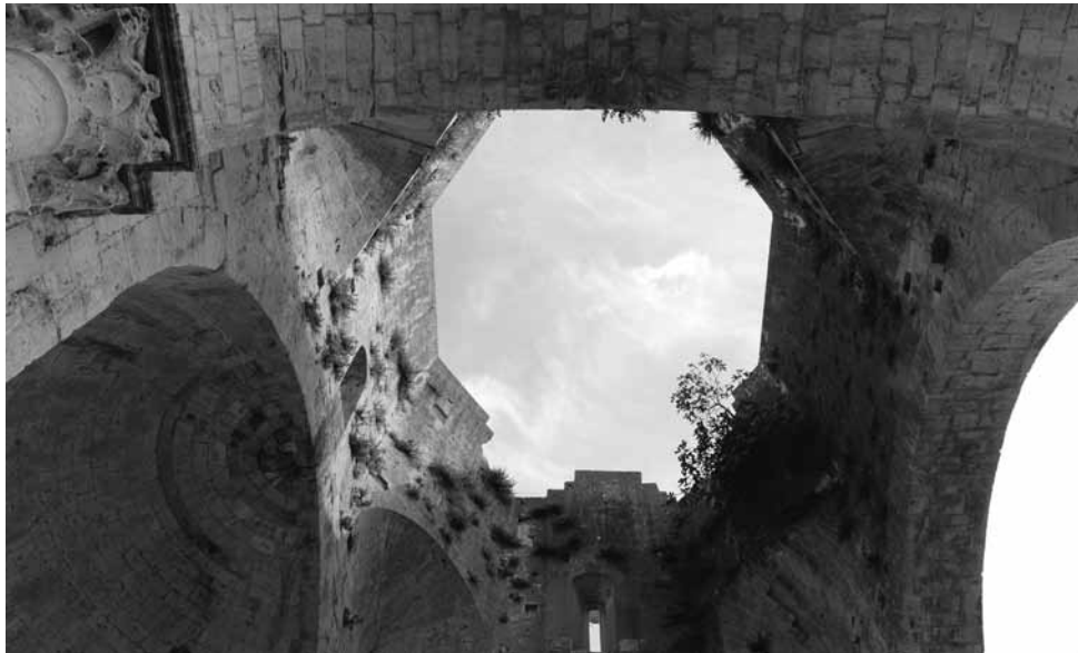
Fig. 2 Bottom view which shows the connection between the presbytery and the base of the cupola. On the left we see the semi-spherical basin of the apse with stereotomic value.
