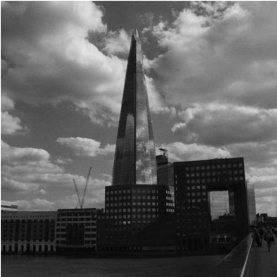
Fig. 4 The uniquely shaped form of the building has become a landmark and a new icon of London.
