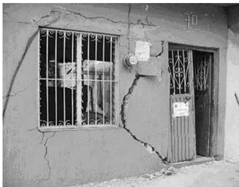
Fig. 1 Behavior of masonry housing under the effect of an earthquake (CENAPRED, 2009).
