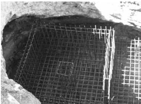
Fig. 4 Chama mosque: the ancient cistern (probably dating to the Roman period) about to be filled with reinforced concrete.
