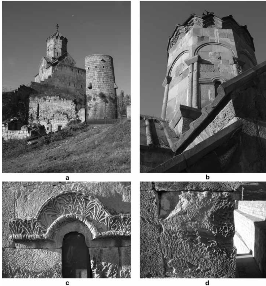
2) a - IX century annexe to Tatev Monastery Complex destroyed by earthquake b - The restored in XX century dome of the Blessed Virgin church of the Tatev Monastery Complex c - "Self-sputtering" destructions and mosses of ancient ornamented stones belonging to basalt group d - Structural transformations and cut off layers from the stone belonging to basalt group
