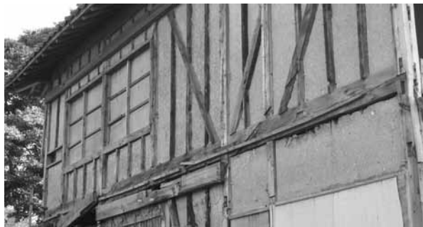
Fig. 4 Aikawa. Traditional house realized with wood and earth, a construction method still in use (O.N. 2014).
