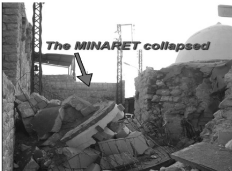
Fig. 3 Chama mosque: the collapsed minaret.
