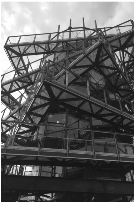
Fig. 1 The blast furnace No.1 extension.
