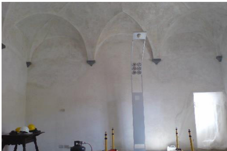
Figure 4: a),b): Building 4, hall at the ground level, photo(left) and IRT mosaic (right) of the northern side. Heating of 8°C in one hour. The picture shows an infilling brick wall in the middle of the structure(solid stone masonry)
