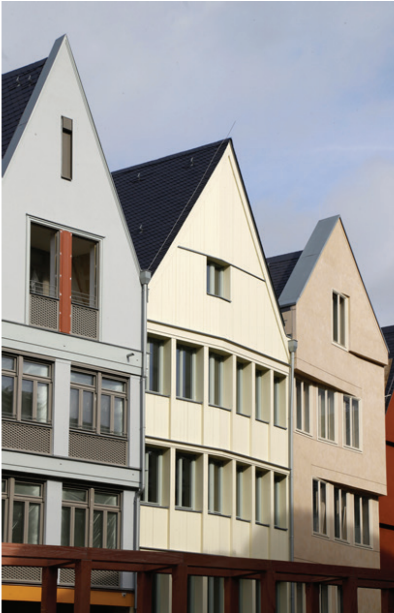
Figure 2: Building re-building at Dom Römer quarter in Frankfurt. The row houses of the side South (in the middle the wooden house by Francesco Collotti with Worzewski, Fantin, Acciai, Corrocher-picture Dettmar)
