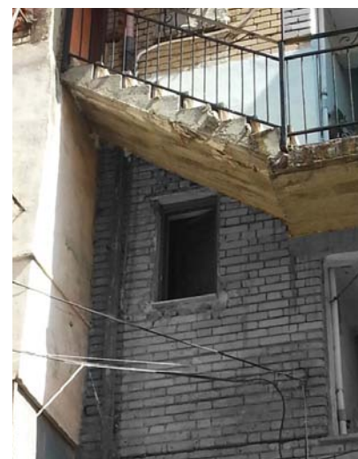
Figure 3: New private stair to an enclosed balcony, between Rr.Ylber Bylykbashi and Rr.Kongresi i Lushnjes-Photo by the authors.
