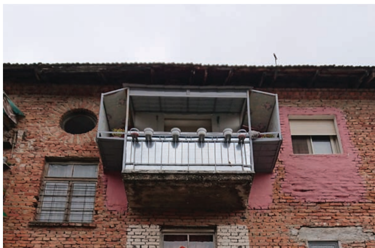
Figure 1: Balcony partially enclosed and expanded in Rr. Komuna e Parisit-Photo by the authors
