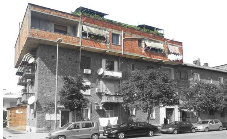
Figure 2: Floor added at the crossroad between Rr. Mihal Popi and Rr.Komuna e Parisit - Photo by the authors.
