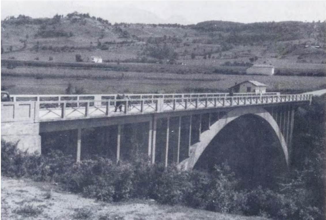
197. Photo of the Gorniqe Bridge.
