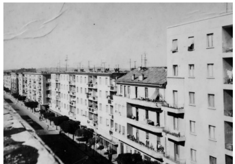
Figure 7 and 8. Durrës Street, Tirana, 1960-1965. Source: AQTN.
