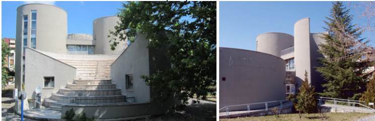
Figure 2. Cultural centre “G. Capograssi” Sulmona (AQ). Source: Photo 2008.
