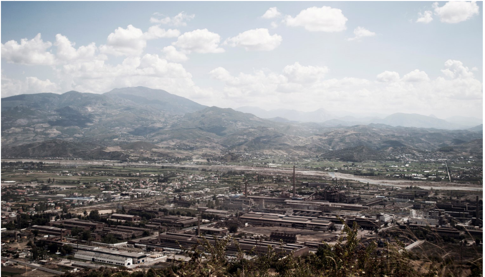
Figure 2.A photograph of the actual condition of the Kombinati Metalugjik in Elbasan. Source: Photo of Marjola Rukaj.
