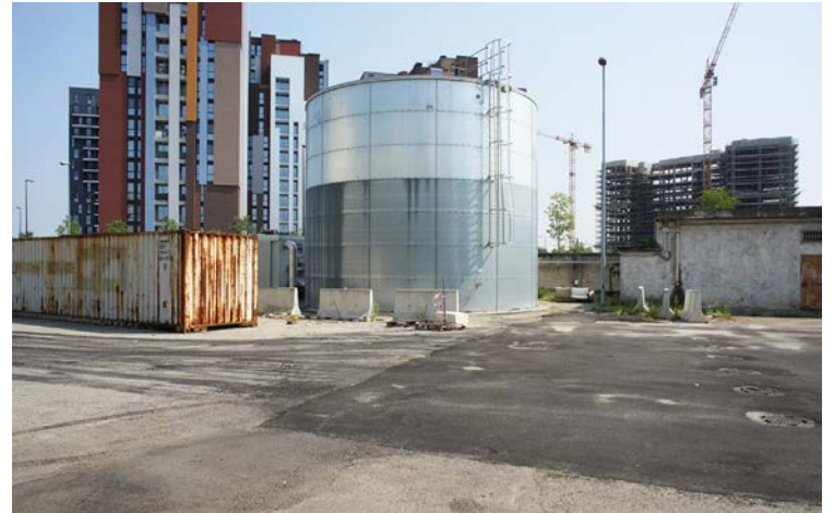
Figure 1. Urban transformation interventions in Milan-Cascina Merlata for an urban island of residential towers.
