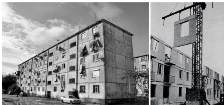
Figure 10. Prefabricated Camus system, built-in Albania from 1971. Source: Wikipedia.
