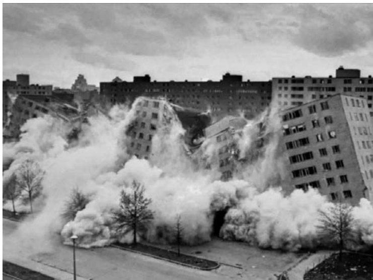
Figure 2. Destruction of Pruitt-Igoe - Source: Minoru Yamasaki.
