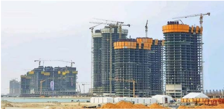
Figure 5. New Alamein city waterfront under construction towers [6]
