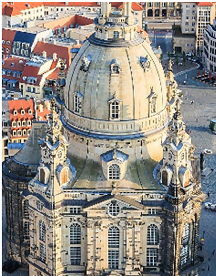
Figure 6. Frauenkirche Dresden – With dark colour we can clearly distinguish the stones reused from the destroyed church. Source: Llazar Kumaraku by Google 3D Map.
