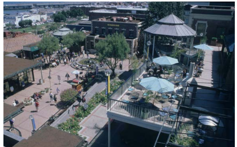
Figures 5. The internal view of Ghirardelli Square. Source: Author's archive, 2008.
