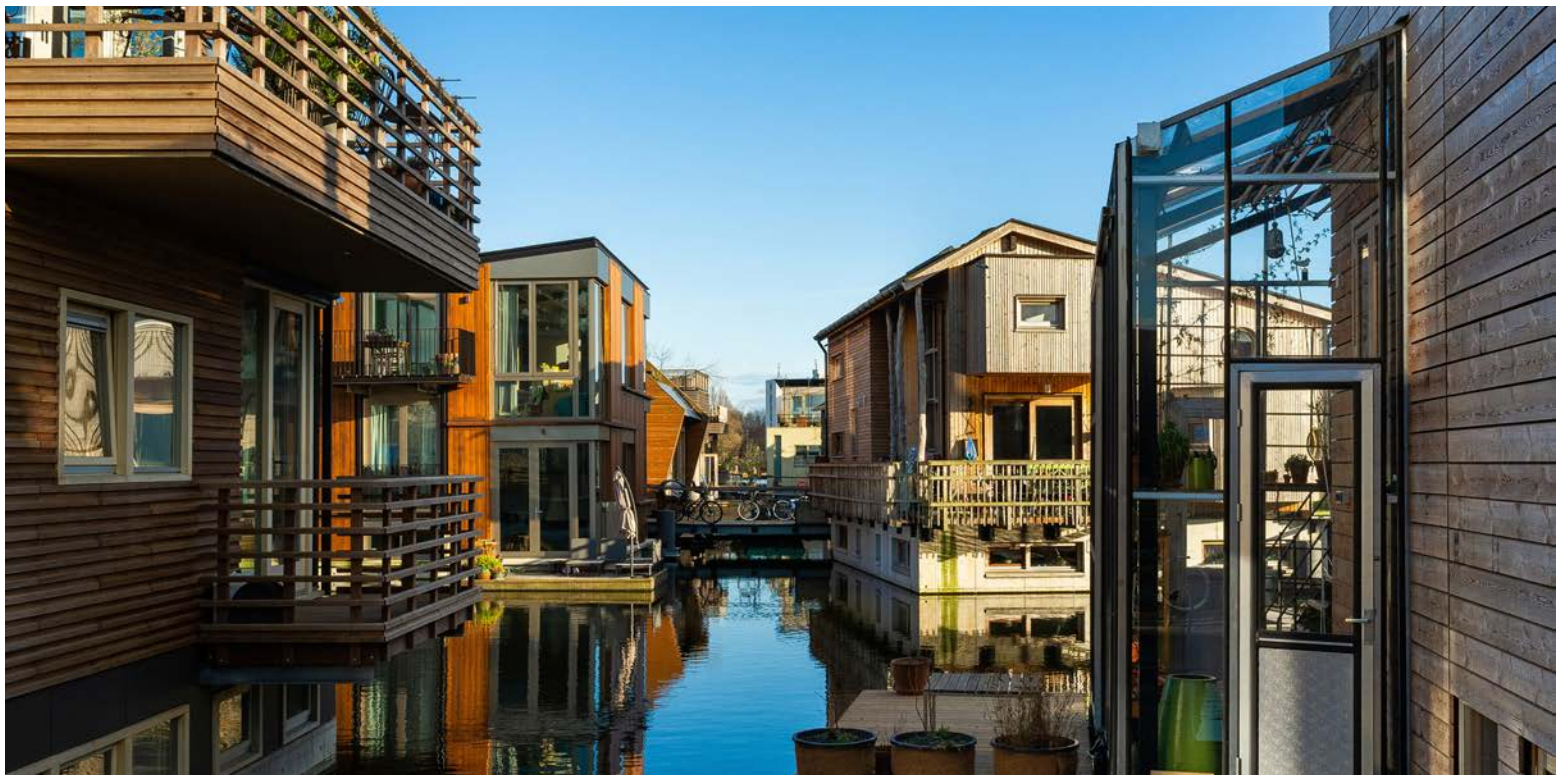
Figure 5. View towards the floating neighbourhoods Schoonschip in Buiksloterham district in Amsterdam. Source: Agnieszka Kurowska.
