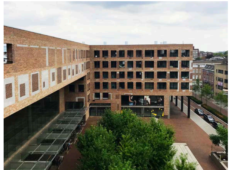
Figure 3. View towards the residential part of the Breda Centraal station building. On the left there is a car park on the roof, under it there are train and bus platforms. Source: Author.
