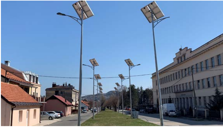
Figure 3. Solar street-lighting in the Boulevard of Montenegro Heroes, Cetinje, Montenegro (photo G. Radović) Tirana (Albania)
