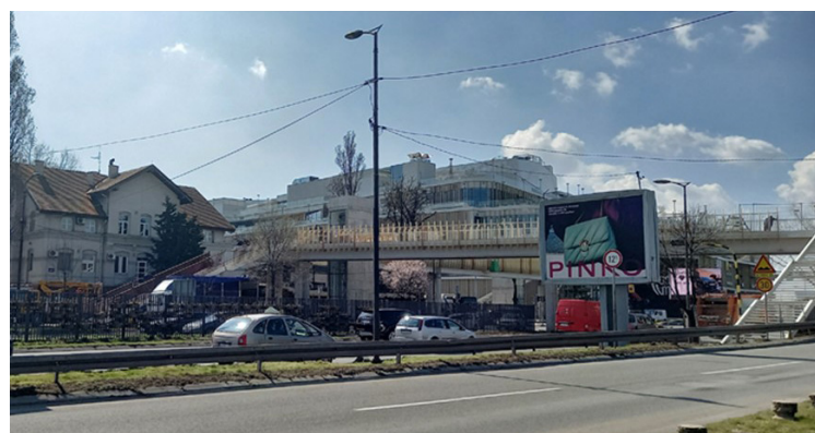
Figure 3. Newly built walkway in front of one of the valued buildings of Sugar factory. Source: Dimitrijević Marković, Pucar.
