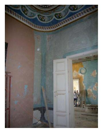
Figure 6. Room with colored finishing plaster of the Ottoman period.
