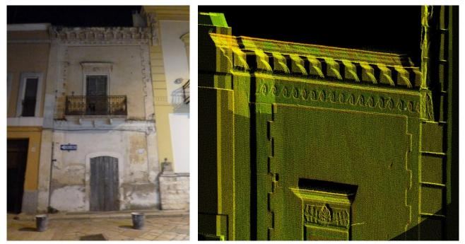
Fig. 7: Carbonara. The small palace in Corso Vittorio Emanuele: the facade and a detail of this by laser scanning.
