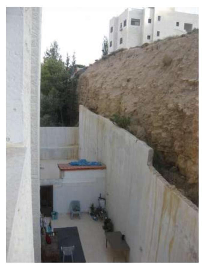
Fig. 10: Retaining Walls on Severely Cut Slopes.
