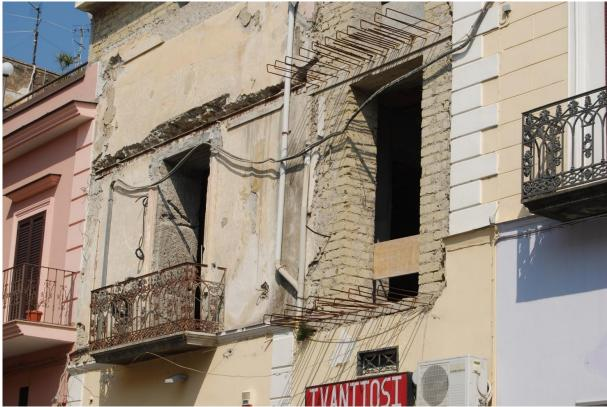
Fig. 2: Sarno (SA), inner-city. Still today it's ordinary to substitute "traditional" building components with incompatible materials and features.
