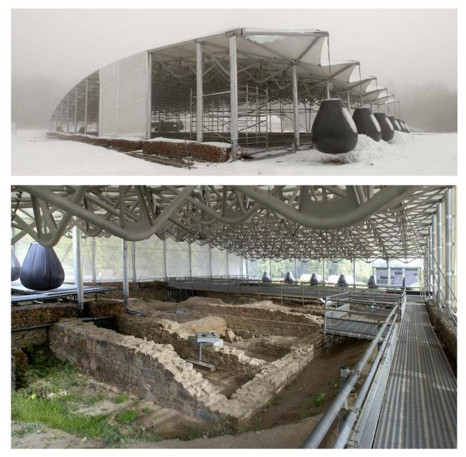
Fig. 10: The shelter designed to protect an area of architectural remains of major importance – those of a mid-1<sup>st</sup> c. BC forum – built without foundation and made of a frame whose pieces weigh only 42 kg each (architect: Paul Andreu ; Antoine Maillier ©Bibracte)
