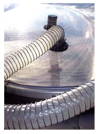
Fig. 13: Villa Nurbs. Aerial view [28] Fig. 14: Detail of the roof 'pillows', showing ducts that regulate solar penetration by inflation and deflation. [29]
