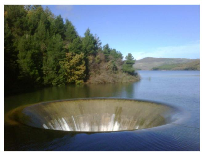
Fig. 1: View of an overflow in full-water condition.
