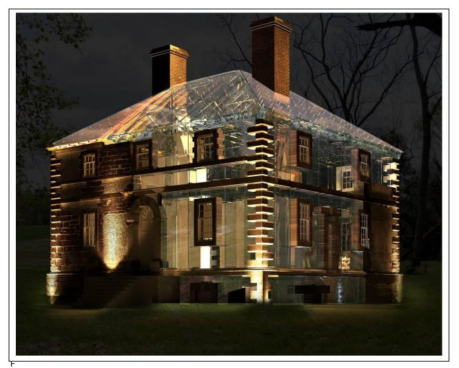
Fig 3: Menokin reassembled with glass providing the structure and fill (Computer rendering by Declan Nevin)
