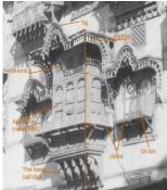
Fig. 4. The roshān construction parts. Makkah 1980s
