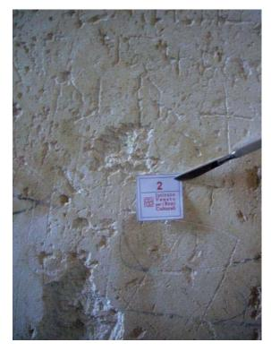
Figure 3. Sampling point 2: finishing plaster placed inside, Ottoman period.
