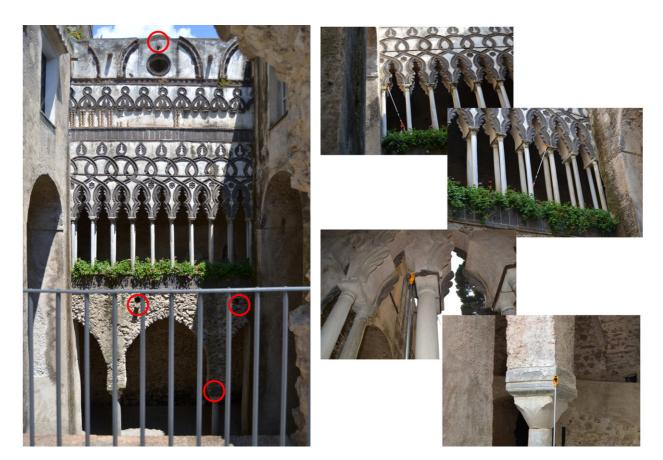
Fig. 5: Recognition which points in the points cloud corresponded to the same points in the topographic network
