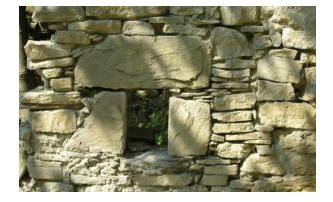
Fig. 6: A window with monolithic frames
