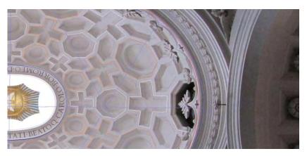
Fig. 1: Photo of the dome (C. Falcolini) and overlay of the photogrammetric restitution and geometric construction of the "canonical oval"
