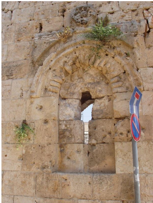
Fig. 5: Stone deterioration and vegetation that took root in an arrow loop, before and after the conservation work.
