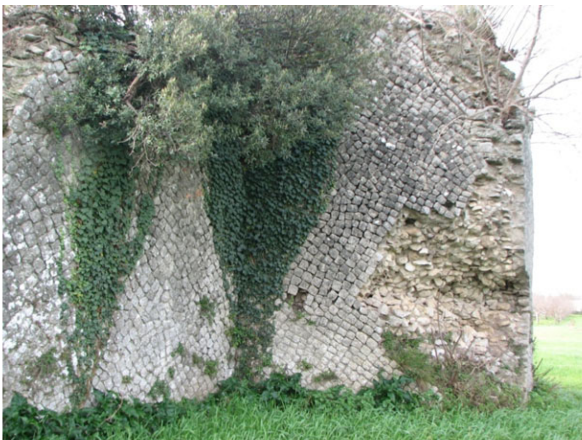
Fig. 2: Detail of insertion hexagonal tower-curtain wall.
