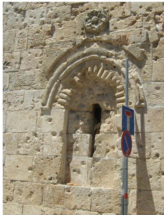
Fig. 5: Stone deterioration and vegetation that took root in an arrow loop, before and after the conservation work.
