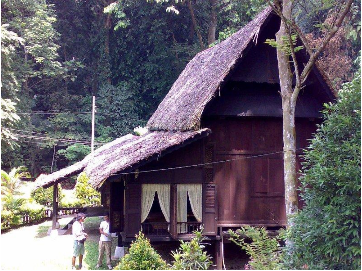
Fig. 1: An authentic Malay house in the Melaka Bumbung Panjang long roof style, with nipah palm attap roofing and tebar layar at the gable ends. The roof space holds an attic floor, which in the old days was used as a bedroom for maidens of the house or to store household assets. Modern buildings using this form can have the water tanks in the roof.
