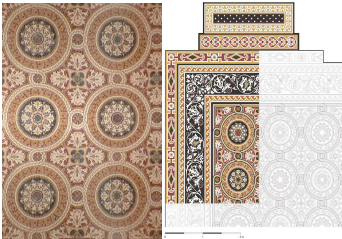
Fig. 11-12: The floor of the Chapel of Pius IX. A) partial image, B) graphic restitution showing how the geometric pattern was developed.
