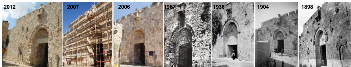
Fig. 4: The Zion Gate façade throughout history, including the conservation work carried out in 2007.
