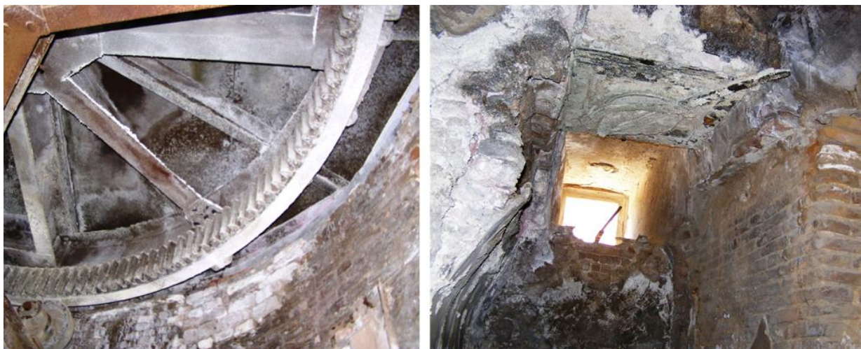
Fig. 8: Polluted material on the furnace wheel (left) and the condensation building (right).
