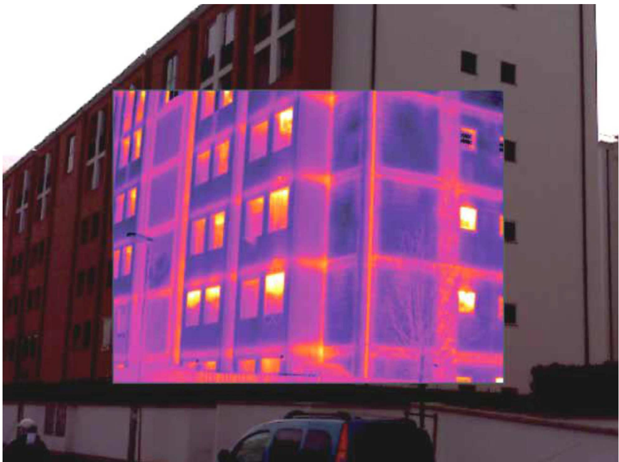
Fig. 8: Firenze, San Lorenzo a Greve, via Tiziano, year 2010. Thermographic analysis of the housing stock for the Italian Legambiente campaign on energy efficiency in buildings (da http://www.legambiente.it/sites/default/files/docs/tuttiinclassaper_sito.pdf ).
