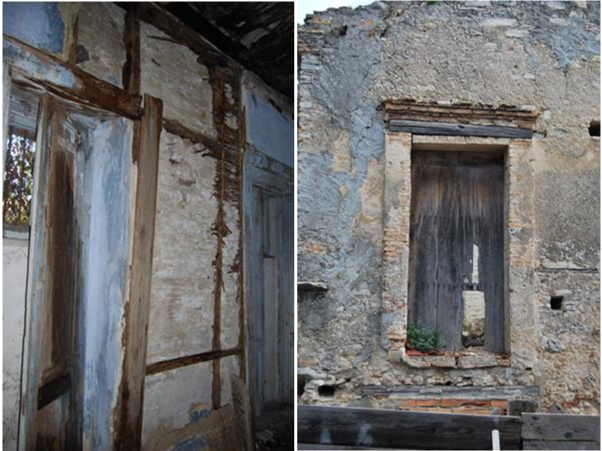
Fig. 1-2: Mileto (VV), the ex-Episcopal Palace. Re-built after the 1783's Calabrian earthquake the fabric adopted a chestnut timber framework with inner coating of rendered "wattle and daub" technique.
