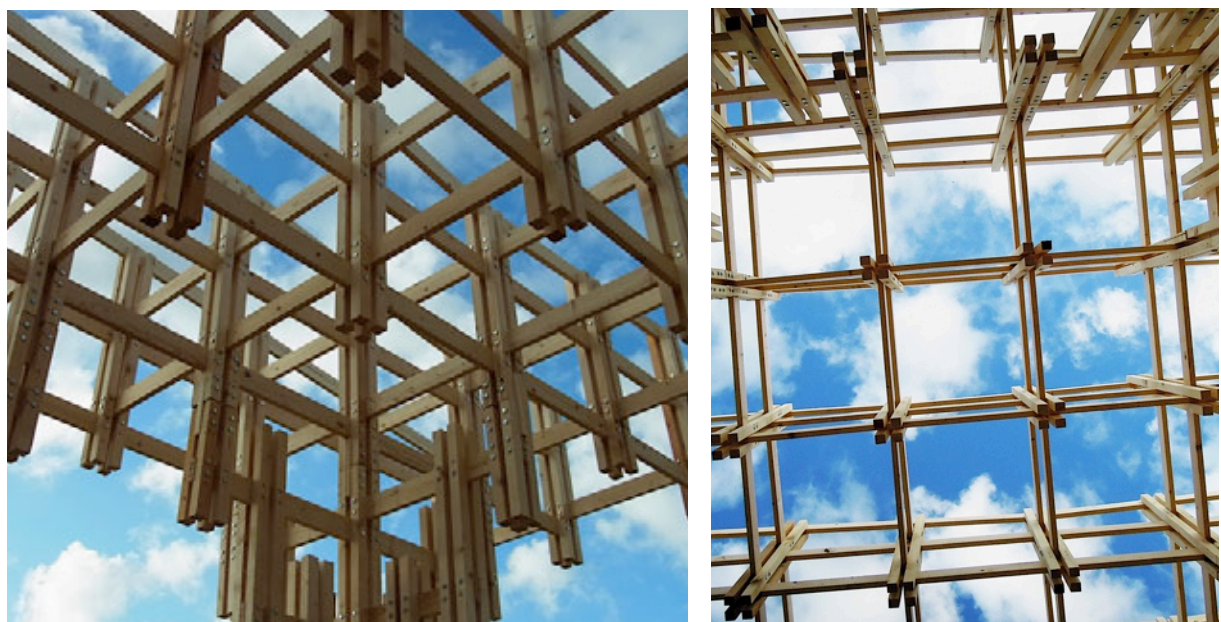
Fig. 9: The whole structure of the shelter is made by a joint system of 4 small struts bind by x-y direction beams with M6 screws. The screws add on resistance against rotational movements due to horizontal external forces.
