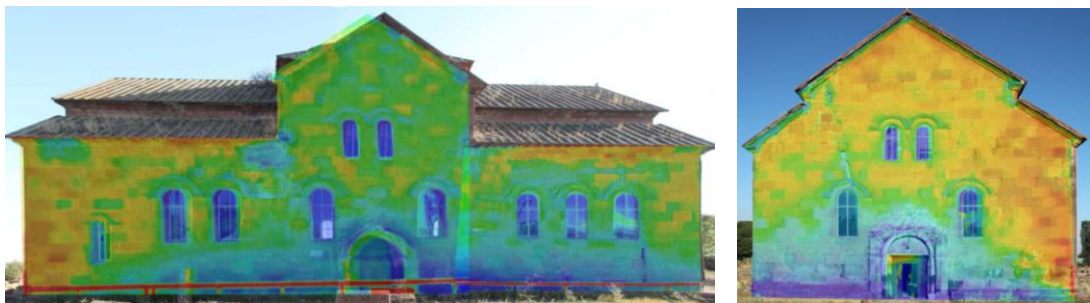
Fig. 10: The thermography applied to the walls has provided significant information about the masonry
