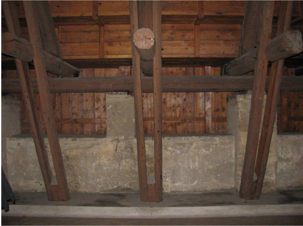
Fig. 5: A view of the load-bearing structures under the bleachers.
