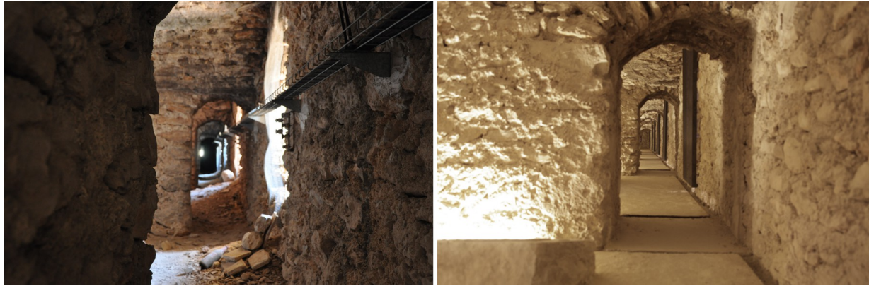
Fig. 4: (Left) The ambulatory prior to the intervention. It was unpaved and the upper surface of the lower vaults can be seen. The wall bears cabling trays and the attachment elements of obsolete facilities, which reduce the space for passage between the buttresses. (Right) The ambulatory after the restoration.
