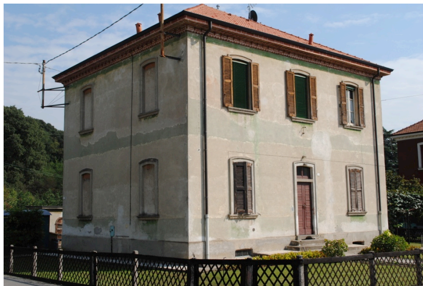
Fig. 6: Residential building; where it has been conserved, the original plasterwork is well attached to the masonry support and the original faded finishing show signs of “noble” deterioration, or rather, a progressive fading of the material that gradually brings out its transparency
