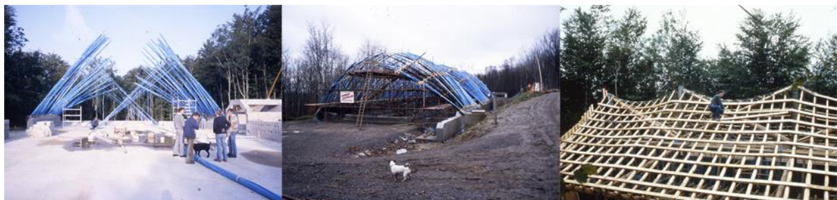
Fig. 11: Building with forestry waste: 1. The workshop building during the bending process 2. The workshop's arches nearing completion 3. The building of the refectory under construction.
