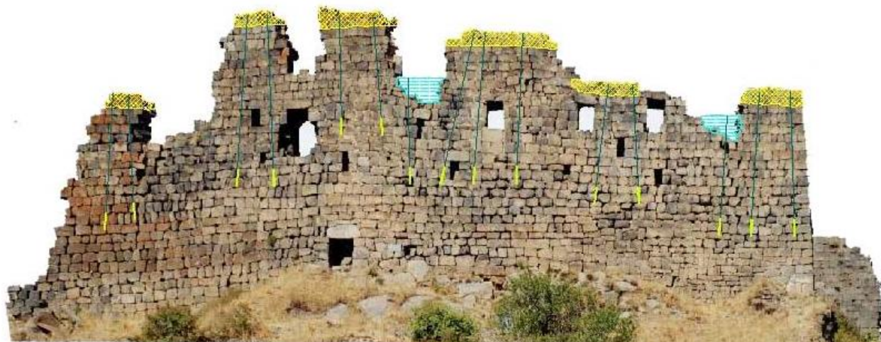
Fig. 4: The consolidation intervention proposed for Anberd castle by adopting steel post-tensioned bars
