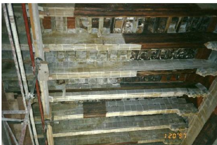
Fig. 13: Intervention to restore a wooden floor.
