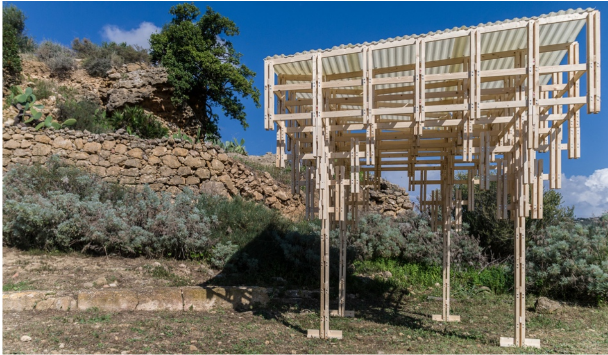
Fig. 8: The Park Agency asked for a shelter with a large roof, designed to carry as far as possible the rain from the excavations, and to minimise the surface area of column base.
