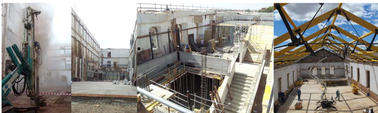
Fig. 6 : LRC construction. From left side to right: foundations, protection of archaeological remains, internal construction and roof.
