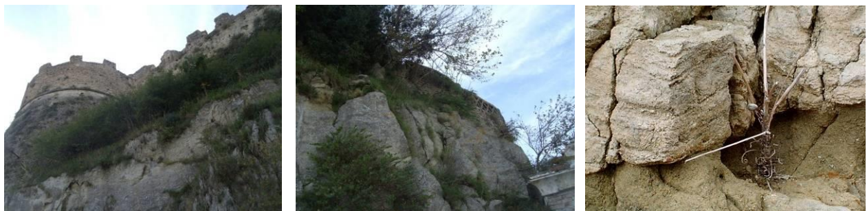
Fig. 5: East side of the castle: biological degradation
