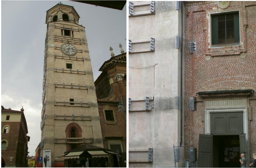
Fig. 2: The bell-tower after the provisional safety measure (2012).
