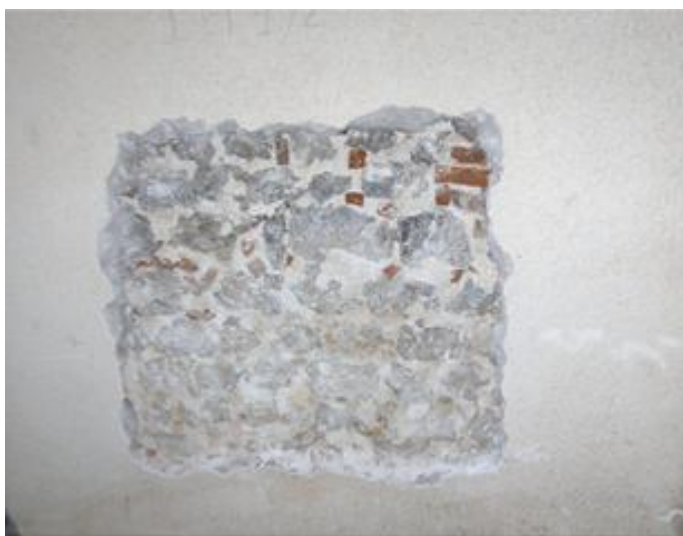
Fig. 1: Typical “Apparecchio Aquilano” masonry wall covered with plaster.
