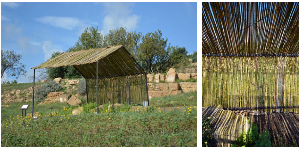
Fig. 13 In order to optimize the structural performances and to minimize the size of the structure, the shelter is made of a 5x5 cm width profile in Corten steel.
