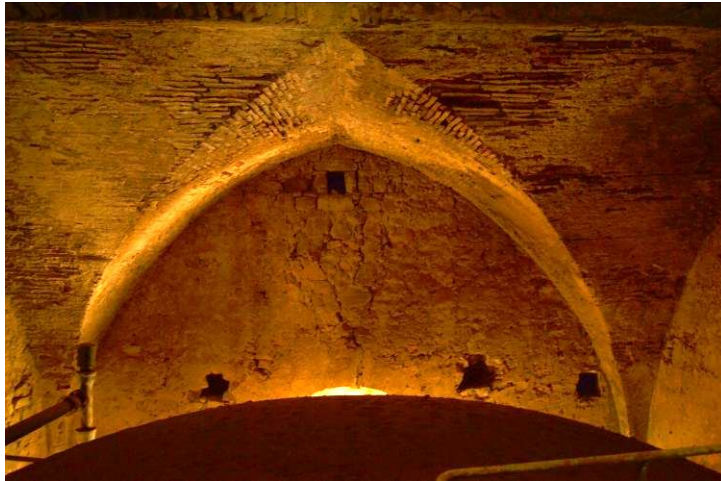
Fig. 4: Inside view of the Normand tower with the cracks on the wall down the vault.
