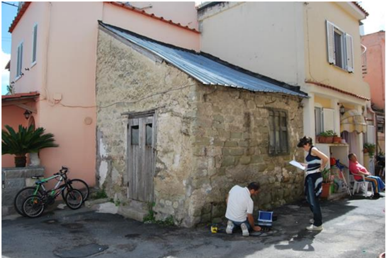
Fig. 4: Ischia. The typical building solution known as “baraccato system” for huts. At the bottom a geo-radar prospections equipment used for timber frames surveying.
