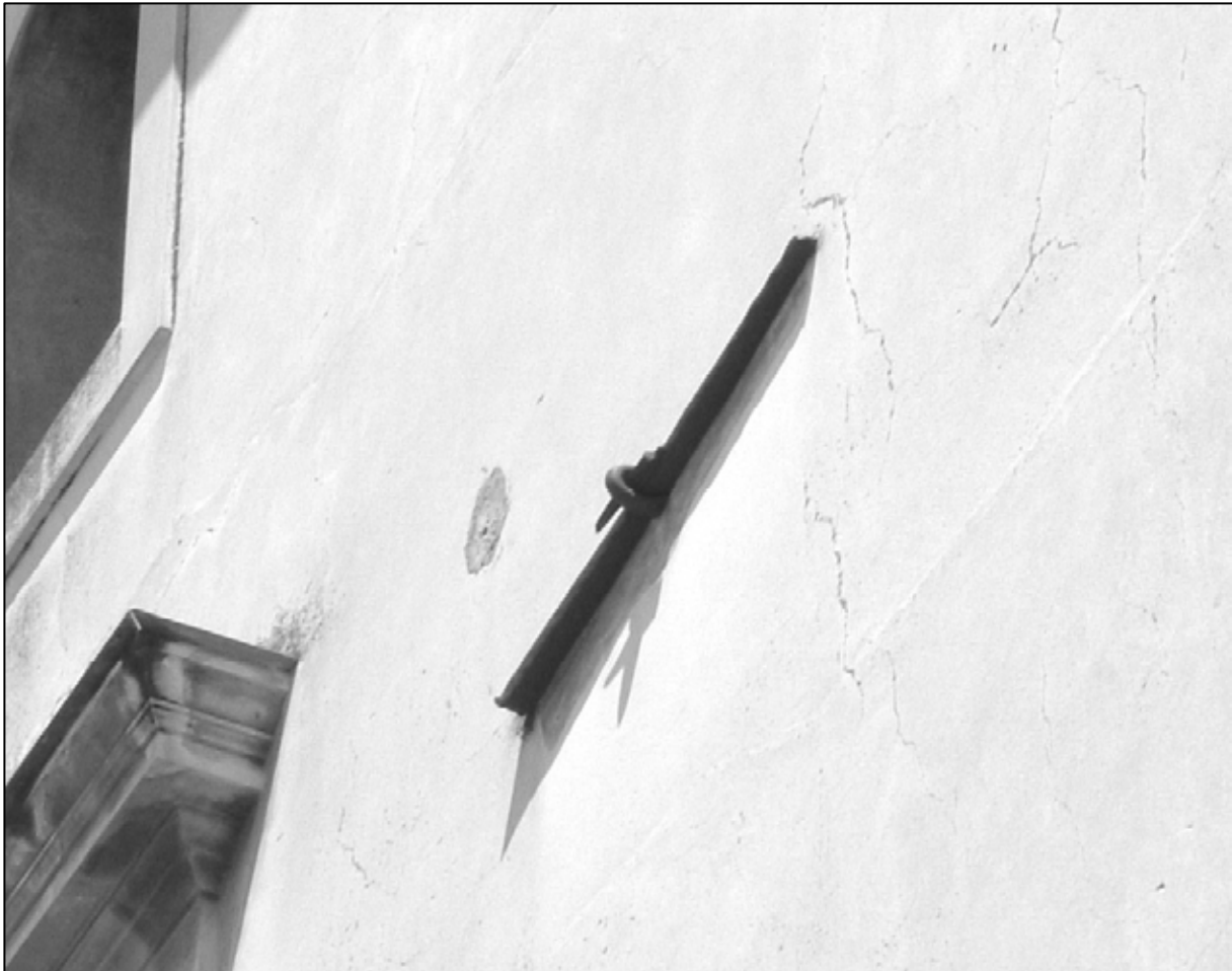
Fig. 5: The anchor made up by an eyelet realized in extremity of the beam or tie-bar and by a little pile. It fixed the little pile into the eyelet and it secured with a wedge. (Residential building in Aversa)
