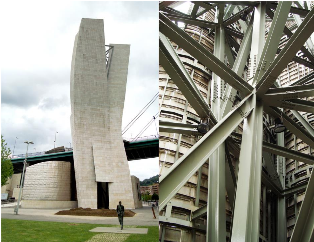
Fig. 5: “the harsh realities of the universal system”: 1. Part of the Guggenheim Bilbao as seen from the exterior. 2. The structure of the above part. Architectural Design by F. Gehry and structural design by Skidmore, Owings & Merrill, 1997
