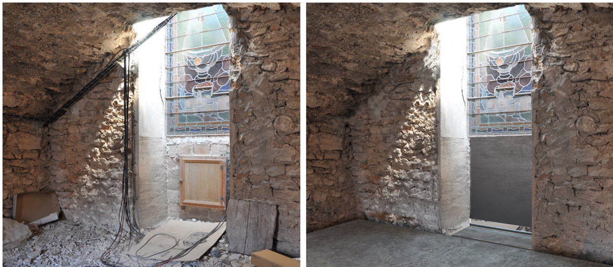
Fig. 3: (Left) Old wooden window used for ventilating the nave, together with the cable duct above the ledge. The window is interrupted by the vault and the ambulatory roof. The lower section of the window was deprived of direct light from the exterior. (Right) Windows after the restoration.
