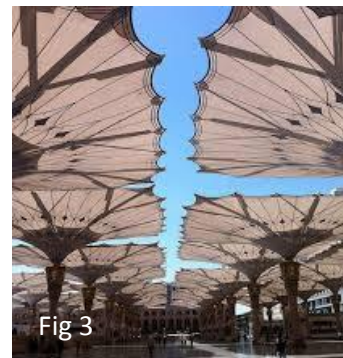
Fig. 3 Shade umbrellas are in place within the pavilions of Mesjid Nebawi. This innovative design allows for a flexibility of space during different types of weather, they are not overbearing in scale or foot-plate and are folded when not needed allowing a clear view-site.
